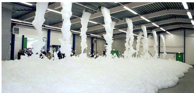
*Picture 2. Foam extinguishing system*
