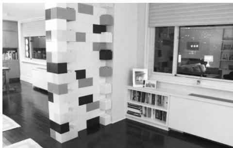
As you can guess, the blocks are connected together by a "spike-groove" principle as constructor LEGO, what allows you to build quickly without using a solution or glue. For the rigidity of the building structure in the central hole of block, which has diameter 110mm, is placed reinforcement and then poured by usual concrete. Because of grooves and ridges in the clutch it gives an effect of insulation.
